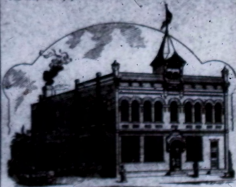
Republican-Register Building, 154 and 156 East Common Street.
